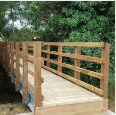
Bridges across small watercourses may be required to ensure inclusive access to strategic routes across the Site. It is recommended that these are timber construction or possibly timber composite in areas prone to flooding, and can often be sourced as 'kits'. Minimum width of 1.8m with balustrade to either side. Image Source Secure-a-Field Ltd.
