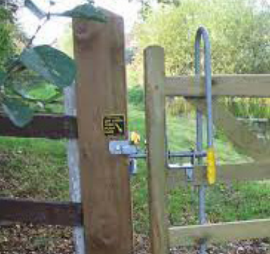
Pedestrian gates: Gated access is recommended over stiles to enable inclusive access to the Site. D-shaped handles to enable latch to be opened with one hand and allow for increased manoeuvrability. Image Source: Centrewire.
