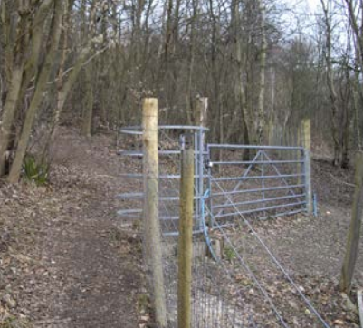
Metal access control kissing gate and field gate with timber posts at Site perimeter where stock-proof fencing is present Image Source: Paul Farmer CC BY-SA 2.0.
