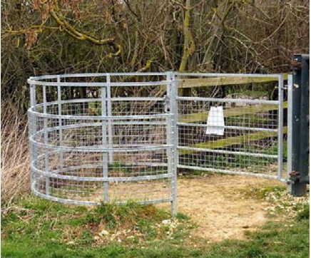
Pedestrian gates: Kissing gates with larger access and turning circles for limited mobility and pushchair access. Image Source: Steve Daniels CC-BY-SA-2.0.
