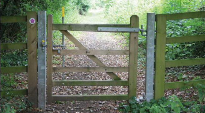
Equestrian gates: Latch release, operated with one hand. Latch on the top of the gate so that the rider may not have to dismount. Image Credit: Centrewire.
