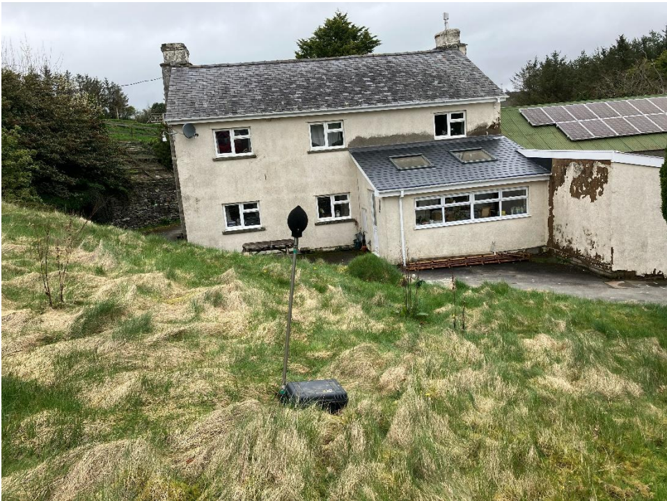
Figure C7 - View of the monitoring location at Pen y Banc looking east
